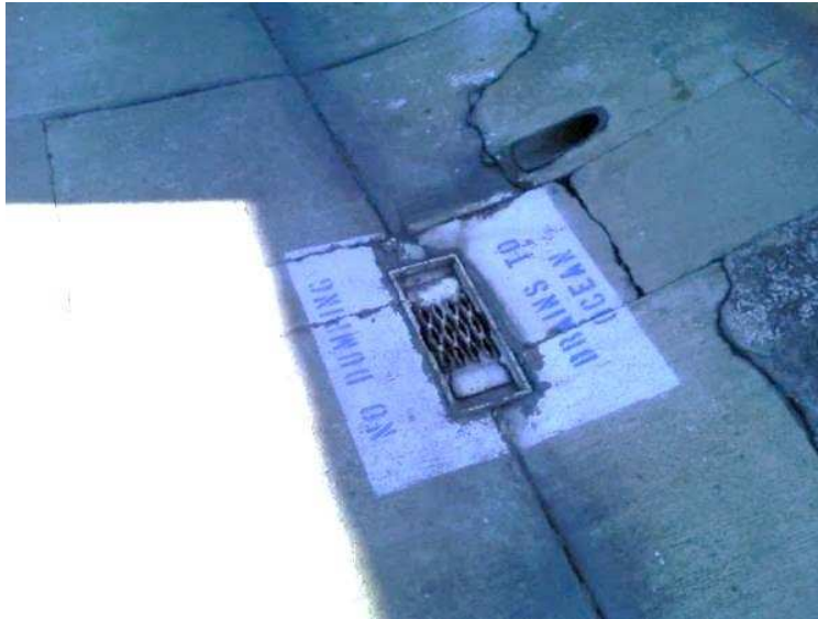
Figure 5. Windward Catch Basin Stenciling
