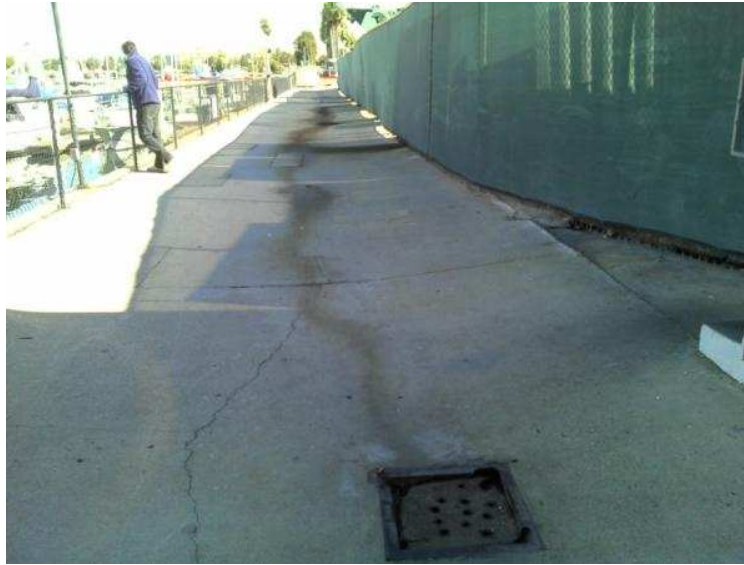
Figure 9. Example Catch Basin at The BoatYard
