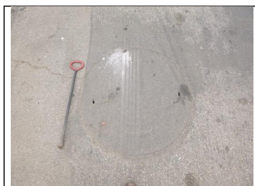
Figure B-4. Currently No Safe Access to Former Watershed Station MdR-2
