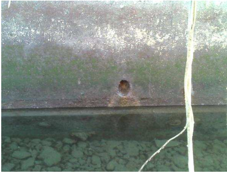
Figure 7. Outfall Adjacent to The BoatYard
