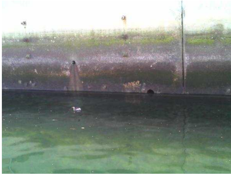
Figure 3. Example Outfall at Windward
